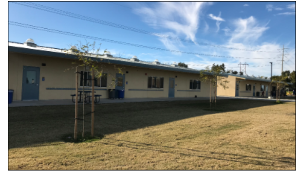
New Building Addition
